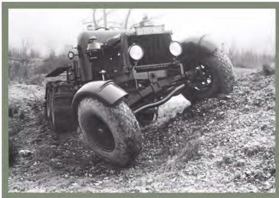
● Early R100 artillery tractor chassis doing what it does best during trials at Watford. Note the tracks enclosing the rear wheels.
