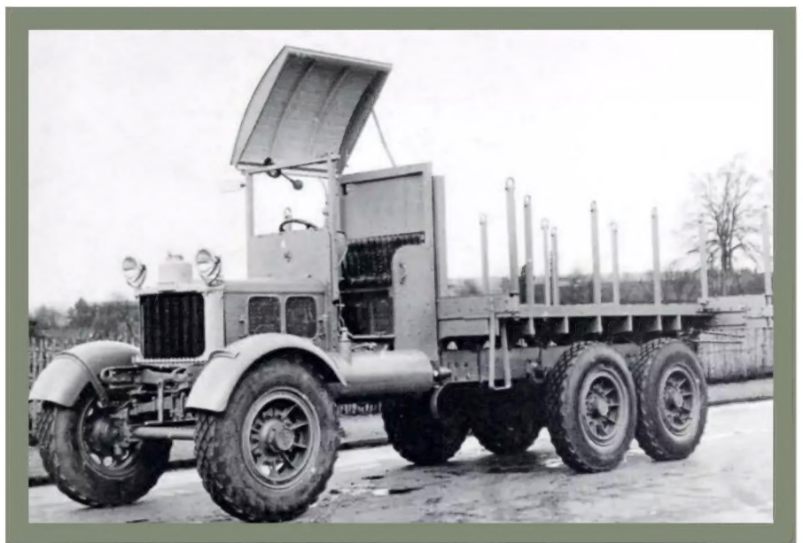
● Another shot of one of the two trucks sent to Venezuela for oilfield work showing the narrow, one-man cab that allowed pipe sections to be carried on either side, thus effectively extending the load platform without extending the truck. The cast wheels were a feature of Pioneers until the mid-thirties.
