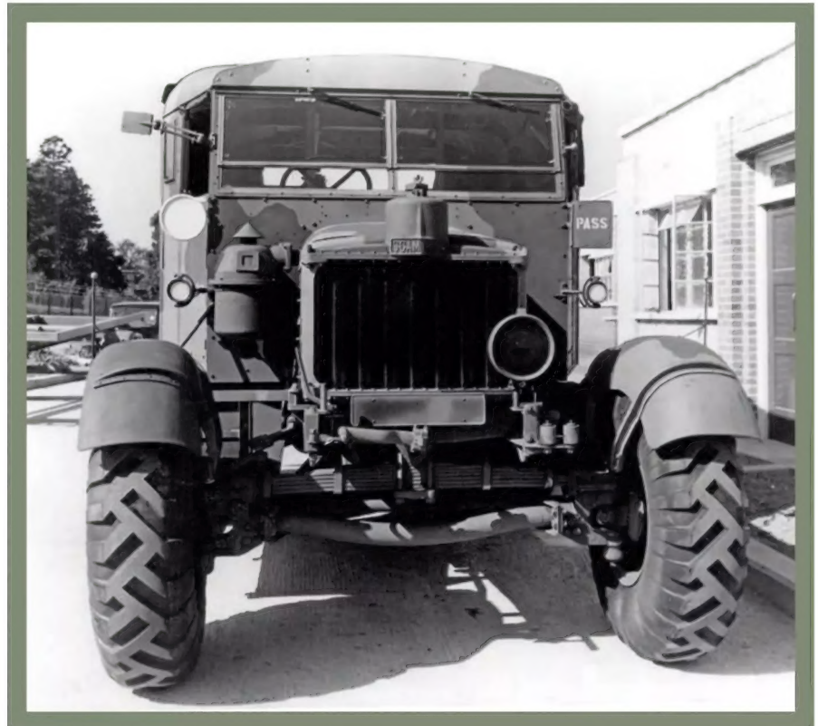
● The looming, friendly presence of the iconic Pioneer... captured at Scammell's Watford works. The two-tone camouflage, and the fact that the name 'Scammell' is cast into the radiator header, tells us that this is an early production vehicle, probably photographed in 1940.
