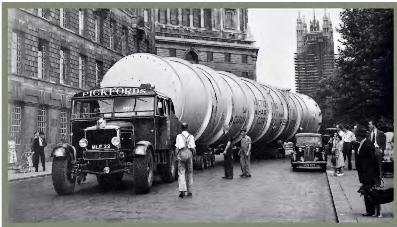
● A Pickfords' Pioneer 80 threading a massive fractionating column through central London.
