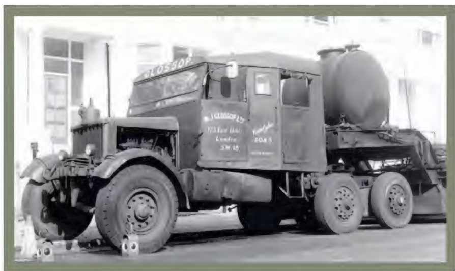
● Another road-making tractor belonging to Glossops, this one looking slightly battered and under-shod with its single rear tyres. Note the huge fuel tank mounted over the fifth wheel.
